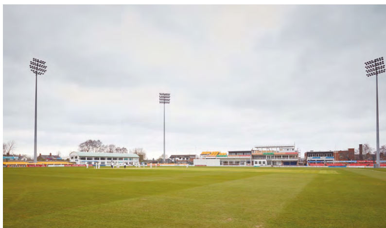
Let there be lights: the ICC-standard floodlights at the Fischer County Ground at Grace Road
